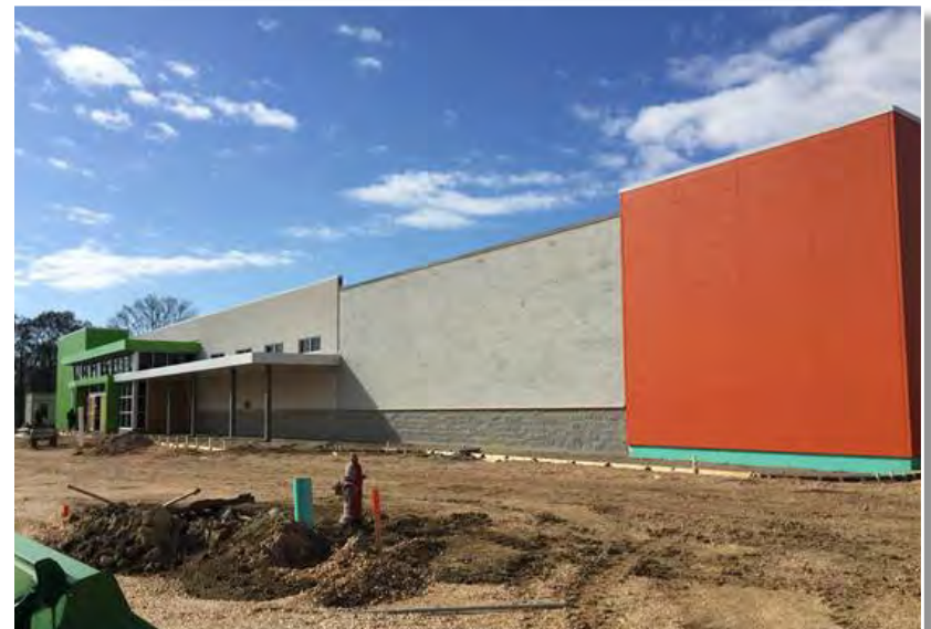
Construction Photos: January 2017
